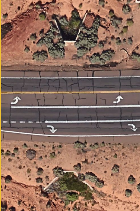
Figure 6: SB US 89 Culvert
